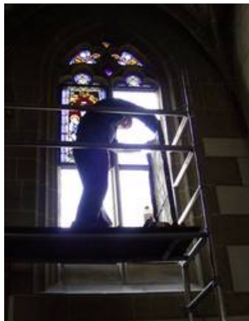
Careful visual examination of the exterior protective glazing prior to the assembly of the conserved medieval glass paintings.
