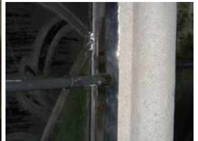
The tap wrench is attached with straps (friction-locked) on the brass frame.
