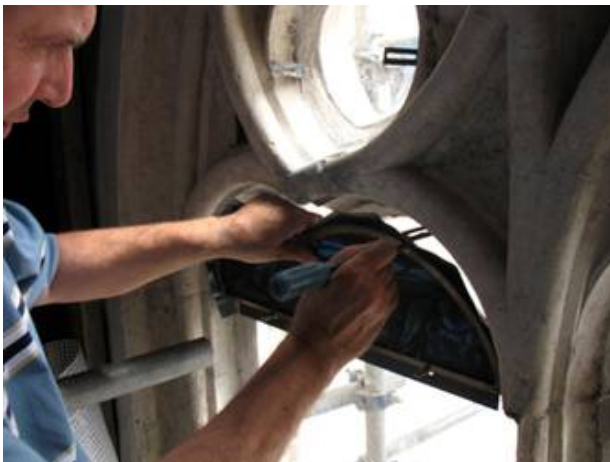
Installation of a header pane into the restraint structure.
