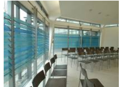
Kreiskrankenhaus (County Hospital) Mosbach, blinds featuring glass lamellae with digital direct printing
