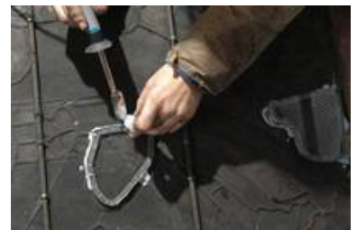
Temporary paint-layer preservation – coverage of loose paint-layer slabs
