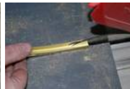
Cutting out of the base if the brass U-profile to avoid gaps
