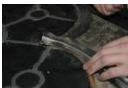
Fitting of the rolled-lead cover
