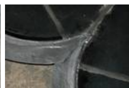
Detail of the finished rolled-lead cover"
