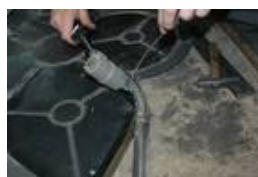
Soldering on (rolled-lead cover)
