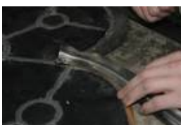
Fitting of the rolled-lead cover
