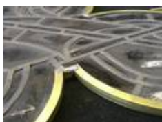
Attention to the smallest detail, brass U-profile and no gaps
