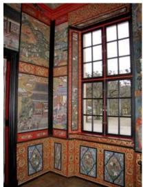
The valuable wall ornaments are protected in the best way possible by our UV-protective glazing, according to the standard international requirements for museums, with a transmission edge of 1% at 400 nm.
