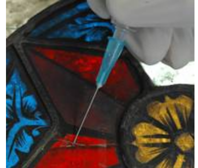
Painstaking handiwork and fine-tuned tools are essential to the adhesion of cracks.
