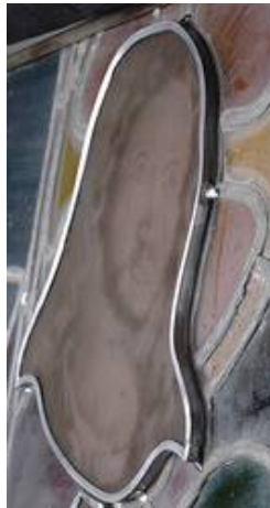
On the rear of the field, a reversibly-applied doubling.
