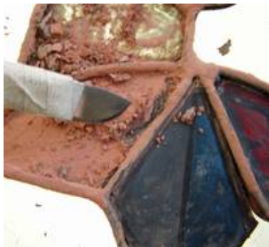
Painstaking exposure of a medieval leaded glass which was covered with wall paint.
