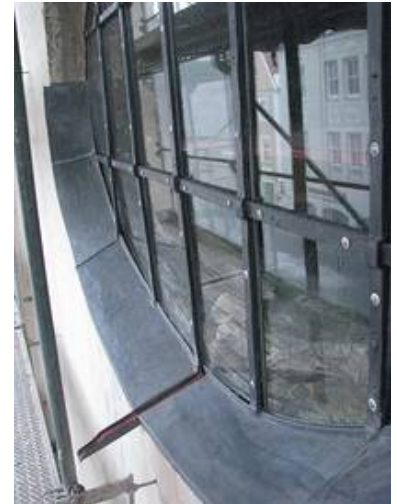
Run-off traces below a church window
