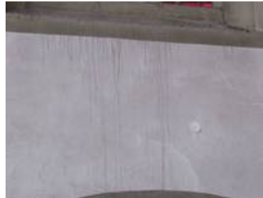
Run-off traces below a church window
