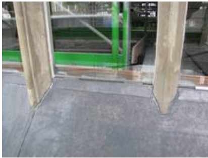
Illustration of a condensate chamfer made of copper and framed by lead on a window ledge covered with lead-sheet panelling.
