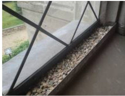
Illustration of a condensation-collector chamfer as an evaporation chamfer on a particularly geographically-exposed structure (which in any event would have been subject to the hazard of water being pressed into the interior due to the prevailing wind pressure).
