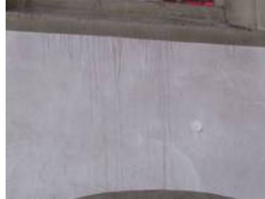
Run-off traces below a church window
