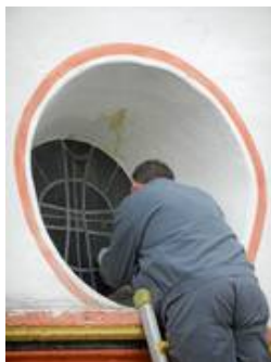
in situ repair of a church window
