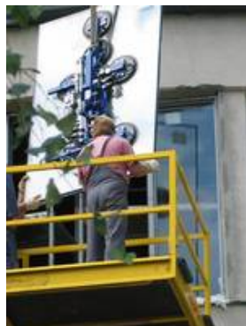
The assembly of the panes took place with a crane
