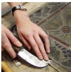
Careful positioning of the lead netting.
