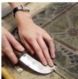
Careful positioning of the lead netting.
