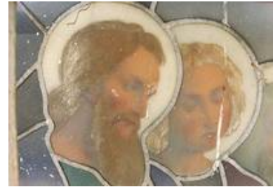
The filigree original lead netting of a glass painting in its previous condition (from the outside).
