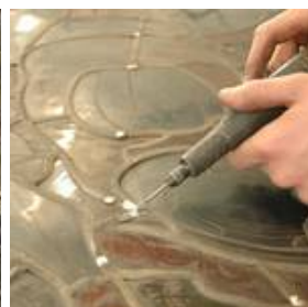
Punctual removal of the lead's oxidation layer.
