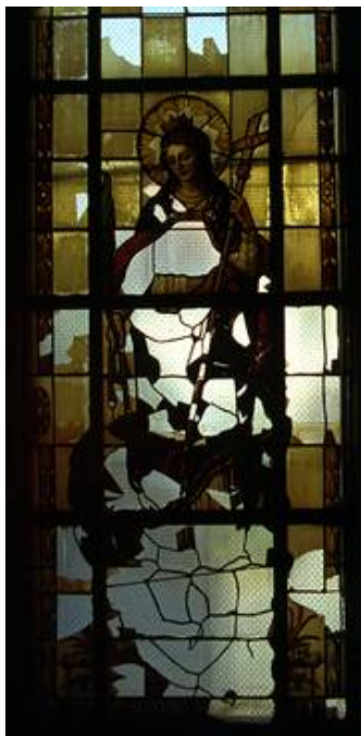
Even this severely damaged lead netting could be preserved in the course of conservation.
