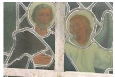
Another window in the same inventory was coated with lead according to the relevant historical specifications. The loss of the filigree character is clearly apparent.
