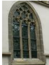
The exterior protective glazing in Bad Wimpfen in its condition after the completion of work
