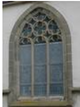
The exterior protective glazing in Bad Wimpfen in its previous condition
